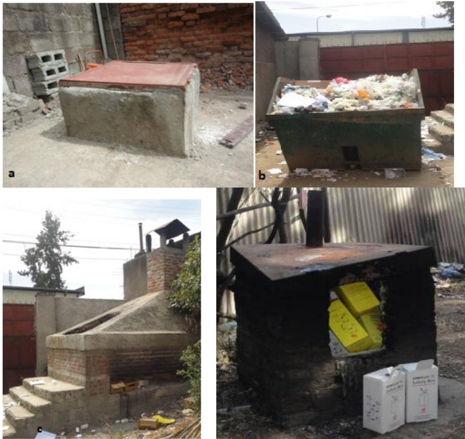
Figure 2 shows the waste disposal system of hospitals (a) placenta pit (b) garbage bin for general waste (c) incinerator for infectious waste and (d) incinerator for needle
